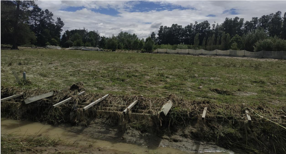
Figure 12 – a fence flattened by the force of water (Wairoa) – such failures can create sudden surges of flood water.
