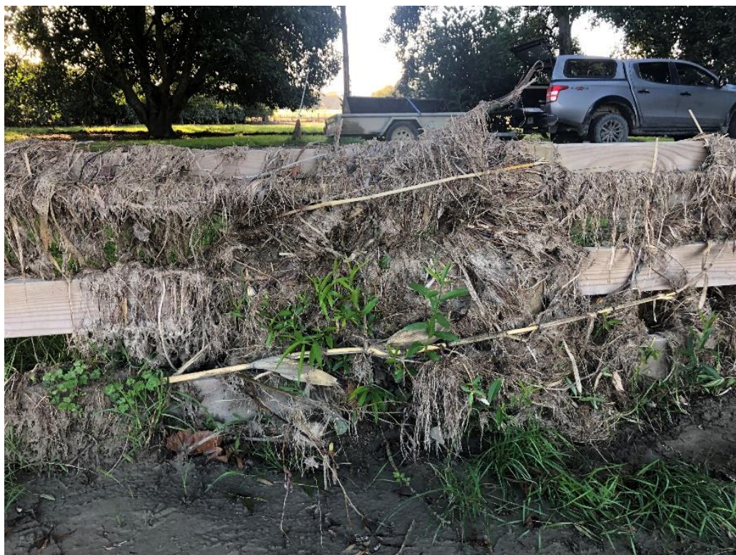
Figure 11 – a fence covered with flood debris or 'wrack' (Wairoa). Such structures can influence how flood waters move through an area.
