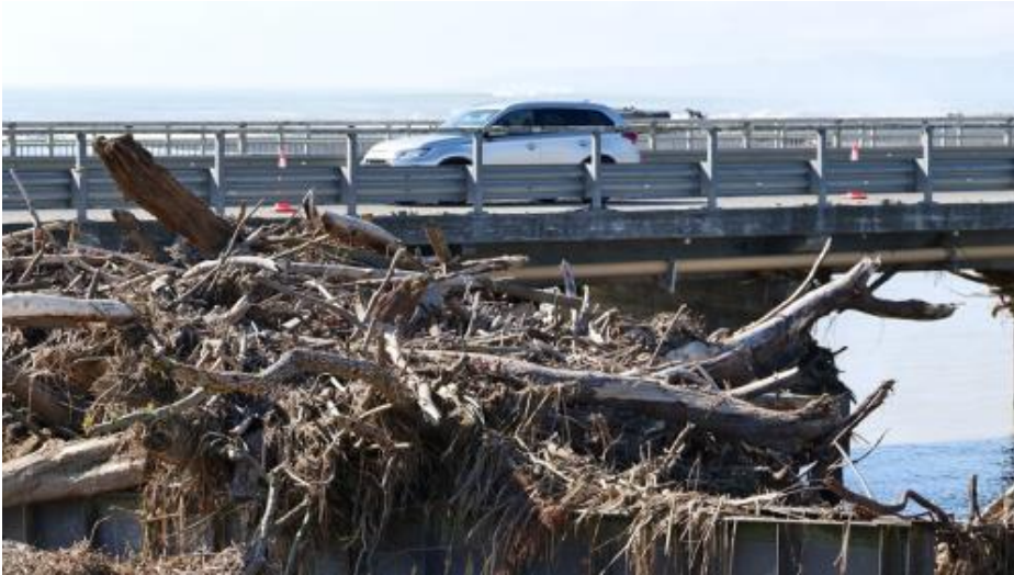
Figure 3 – Awatoto River Bridge, Image courtesy of HBRC
