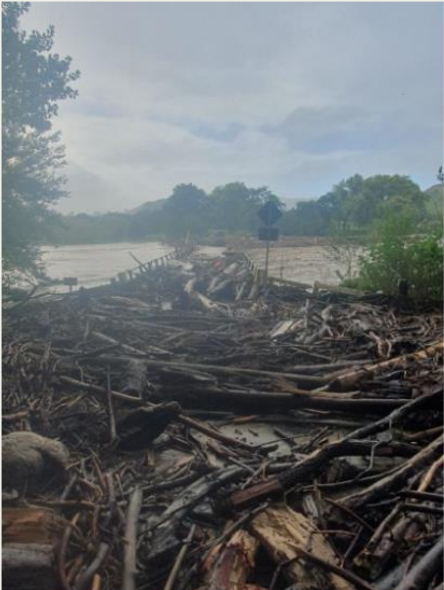
Figure 4 Mixed Woody Debris on Riverina Bridge, Marumaru during Gabrielle – approx. 7 am February 14 2023
