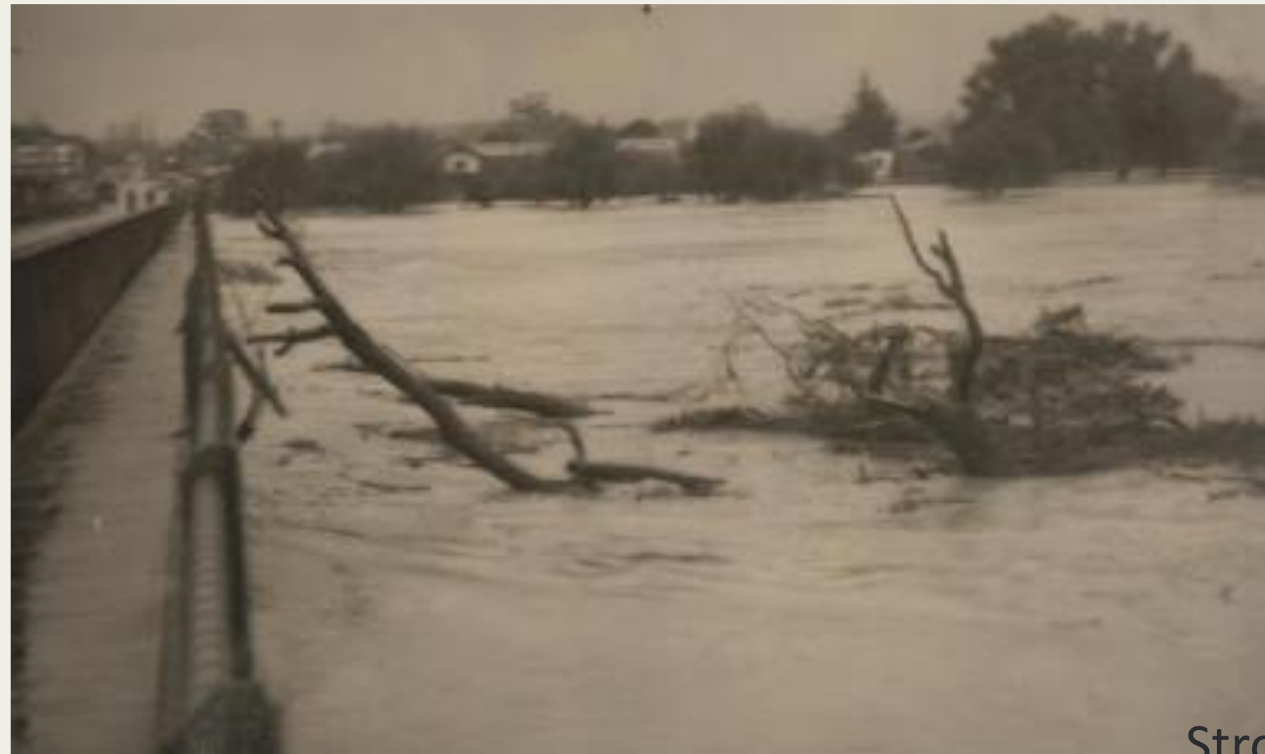
Figure 2 - Woody Debris approaching Wairoa Bridge likely 1948 storm
