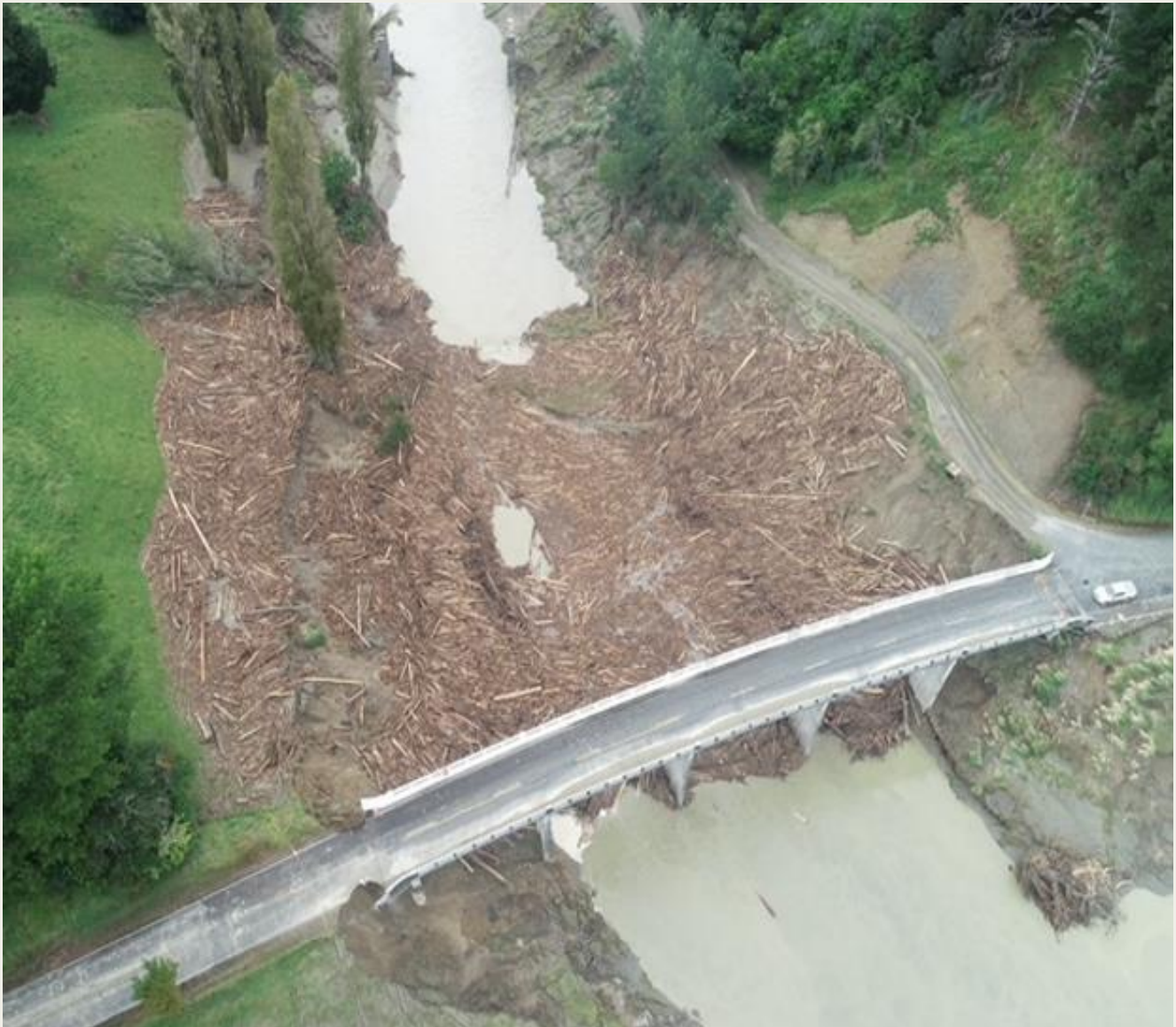
Figure 5 – woody debris behind Kotare Bridge – mainly pine but not physically surveyed
