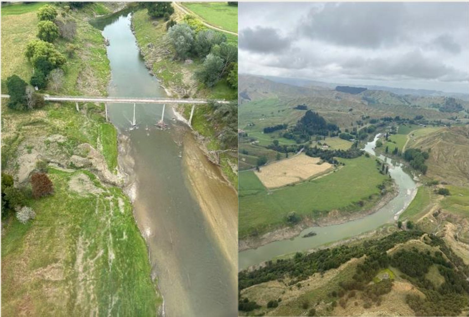
Figures 8 & 9 Wairoa post Gabrielle indicating significant bank scouring.
