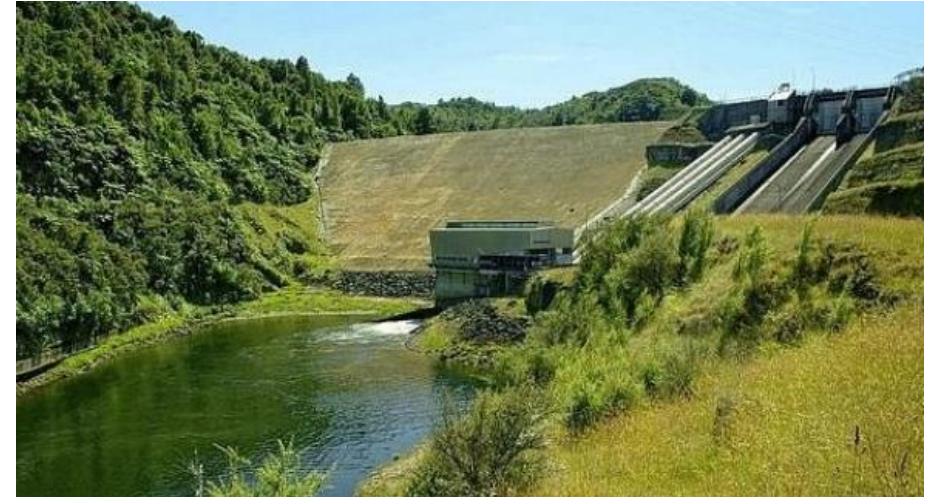
Above: example of the Patea Dam in Taranaki
