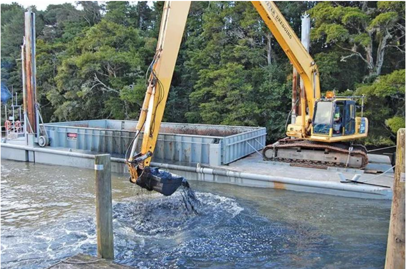
Figure 1: Photo of River Dredging Being Undertaken (Reference 6)
